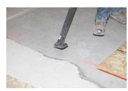
All areas of the renovation space are thoroughly vacuumed with a commercial unit. Removing all dust and debris from the subfloor enhances the bond of the materials to be used later in the project.
