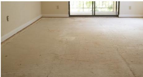
Years of tenant wear have left the subfloors unstable with large amounts of flex that can be felt when traversed.
