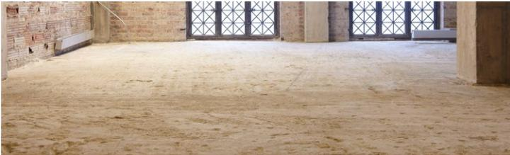
Prior floor coverings, layers of concrete, and dividing walls had been removed leaving a rough concrete surface.
