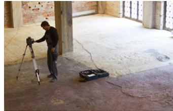
A laser leveling system allowed the installation team to get a more accurate look at the true slope of the floor. Careful measurements and calculations were made to estimate the needed amount of leveling compound.
