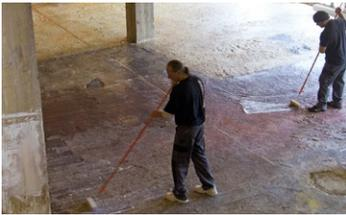
After the concrete substrate was thoroughly vacuumed, the entire surface was primed using Schönox VD, a dilutable acrylic primer that enhances the adhesion between the leveling products and the substrate.
