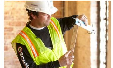
The depth of the gauge rakes to be used in the project are carefully set at the required level. These rakes allow the self-leveling material to be quickly distributed around the project area.
