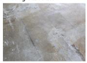
Existing VCT suspected of asbestos content and residual adhesives were present in a number of areas. The project plan called for Schönox products which could cover these areas rather than remove them.
