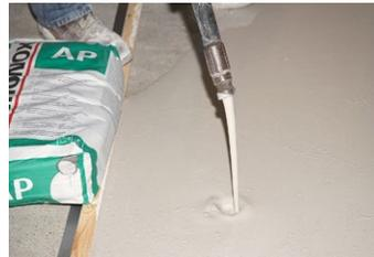
Installation of Schönox AP, synthetic gypsum, self-leveling compound, using a pumping operation, allows installers to efficiently mix product in one location while others distribute the product throughout the area.
