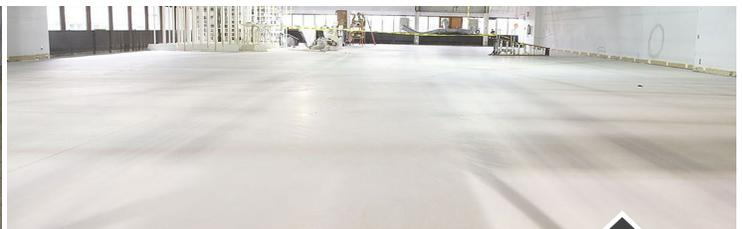
Schönox AP dries to a smooth, white finish ready for flooring installation in roughly 16 hours when poured at a 1/8" depth. The surface is smooth, strong, and even facilitating an efficient floor covering installation to come.
