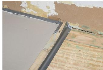
Seams and open spaces surrounding the renovation areas are taped to prevent subfloor materials from flowing into unwanted areas.
