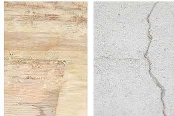
Plywood subfloors at various levels and conditions were throughout the space. A number of substrate areas were brittle or cracked.
