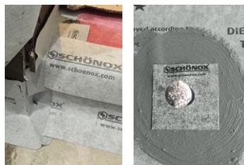
Tighter areas and corners were covered using Schönox waterproofing accessories for inside and outside corners and right angle spaces. Schönox provides pipe cover accessories with 5/8" and 5/16" hole diameters.
