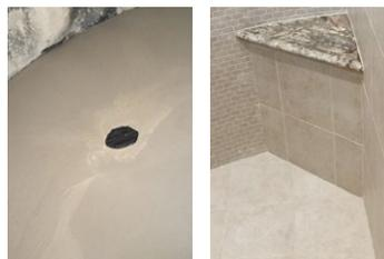
The flow and product characteristics of Schönox US, cement-based, self-leveling compound, make it an ideal material for use in creating a sloping shower floor surface in this irregularly shaped space. Pictured is the shower floor just after Schönox US was poured and the final shower after tile installation.
