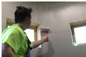
Most substrates were backer board materials. In this half-moon shower, the walls were drywall. Schönox KH Fix, acrylic primer, was applied to reduce the absorbency of the drywall.
