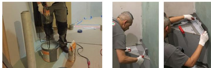
Schönox iFix™, rollable waterproofing sealing adhesive, was used in the shower and bath areas. Schönox iFix™ is solvent free, contains no VOCs, contributes to LEED credits, and uses a special dust-reduced polymer cutting down on those dust clouds so common with other waterproofing materials. Schönox iFix™ was applied to all of the bath areas using rollers that are included with the iFix™ kit. Schönox ST, sealing tape, was applied to this right angle area atop the Schönox iFix™ sealing adhesive.
