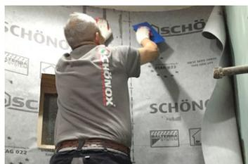
Larger areas of the shower space were covered with Schönox AB, sealing and uncoupling layer material. Schönox iFix™ was used to bond the sealing layers to the surfaces and also to seal the seams of the layers. This process is more than 40% faster than traditional waterproofing methods.
