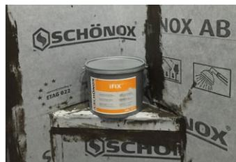
All areas of the shower spaces were covered with iFix™ followed by AB, the sealing layer. AB is made of polyethylene for use with ceramic and natural stone coverings.
