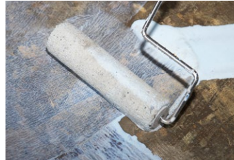
Schönox VD, dilutable acrylic primer, is used to reduce absorption, bind residual dust, and increase adhesion.
