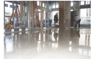
The new subfloor is ready for foot traffic after approximately 4 hours.
