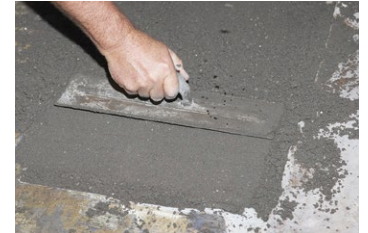
Schönox SEZ Plus, rapid-setting, sand cement screed, is used to repair voids in existing concrete. Ready for covering after approximately 24 to 72 hours.
