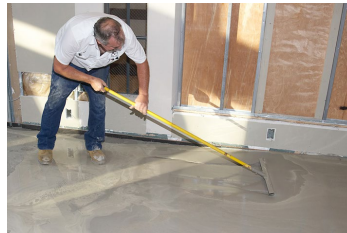
US can be layered in thicknesses above 1/8" up to 3".
