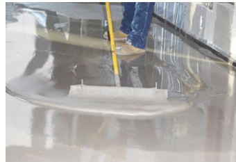
Schönox US mixed with sand aggregate is poured over existing concrete.
