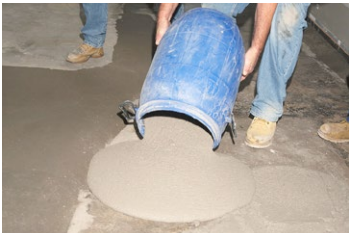
Schönox US, cement-based, self-leveling compound, has compressive strength of 4250 PSI after 28 days.
