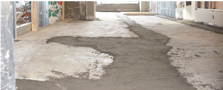
Schönox US, cement-based, self-leveling compound, has compressive strength of 4250 PSI after 28 days.
