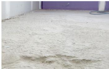
Having undergone an asbestos abatement process, the substrate had residual chemicals within it leading to warranty issues with the proposed new flooring installation. In addition, the concrete subfloor was uneven with pits, valleys, and high spots throughout the space.
