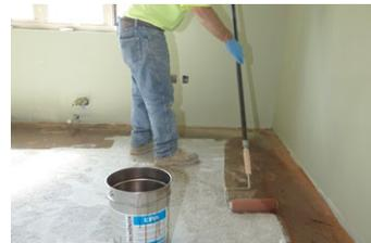
Schönox EPA was applied with rollers directly to the concrete substrate.
