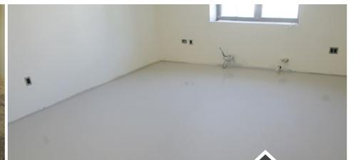
Schönox AP was designed with refurbishment projects in mind allowing subfloors to be covered and renovated rather than demolished with other costly processes. Schönox AP does not shrink or crack. The renovated subfloor will be ready for flooring installation in 24 to 48 hours given the depth of this pour. The tile and adhesive manufacturer fully warranted the new installation after the subfloor process was completed with Schönox products.
