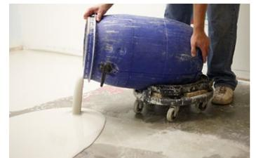
Special dust-reduced properties within Schönox AP keep dust to a minimal level. Created using a by-product of the process used to purify power plant emissions, AP is a strong environmental choice as well as a superior leveling compound.
