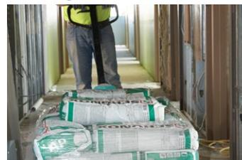
Schönox AP, synthetic gypsum, self-leveling compound, was poured throughout the space providing a smooth surface with a compressive strength of 5800psi. Free of chromates and VOCs, Schönox AP contributes to LEED credits.
