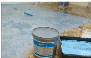
Schönox SHP, ready-mixed acrylic primer, is applied with a roller on top of the Schönox EPA providing a surface that will bond well with the self-leveling compound to be used next. Schönox SHP contains no VOCs and dries in 1 to 2 hours.
