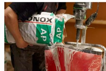
Special dust-reduced properties within Schönox AP, synthetic gypsum, self-leveling compound, allow the product to be mixed inside the facility with a minimal amount of dust.
