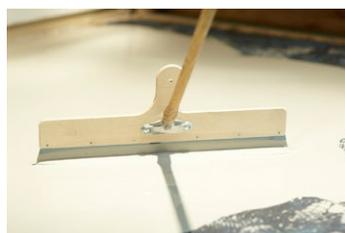
Schönox AP is used to level the entire renovation area. Synthetic gypsum is made from the by-product of the process used to purify emission from power plants making the use of AP a strong environmental choice that contributes to LEED credits.
