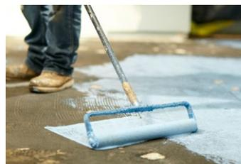
Schönox SHP, ready-mixed acrylic primer, reduces absorption by the substrate, protects sensitive subfloors, and improves adhesion of the leveling compound.
