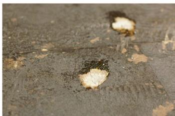
The prior floor covering was removed leaving the exposed concrete and residual cutback adhesive.
