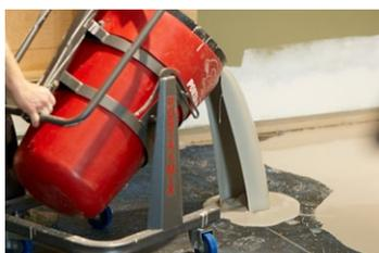
Portable mixing systems allow the efficient preparation of Schönox AP product and easy transport to the pour area.
