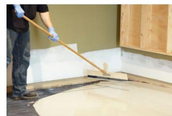
Trowels with extension poles are used to more quickly distribute the leveling compound throughout the renovation space.
