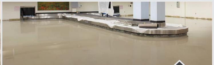
Schönox subfloor products took the baggage claim area from its rough uneven beginning, through the priming and leveling stages, and finally to a smooth strong subfloor ready for floor covering.
