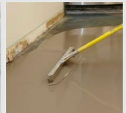
Bags of Schönox ZM, cement-based, self-leveling compound, are pre staged at the renovation area. ZM can be used with both concrete and gypsum substrates. The excellent flow characteristics of Schönox ZM make its pouring and distribution an efficient process. ZM is quickly spread around the renovation area using gauge rakes. With its very low emissions, use of the product even contributes to LEED credits.
