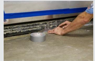
Removing all dust and debris from the subfloor enhances the bond of the materials to be used later in the project. Areas around the base of the baggage claim ramp are taped to prevent leveling compounds from flowing underneath.
