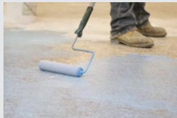
Priming reduces absorption by the substrate, protects sensitive subfloors, binds residual dust, and improves adhesion of the leveling compound.
