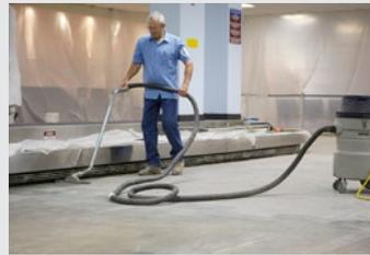
Residual materials not bonded to the substrate surface are removed. All areas of the renovation space are thoroughly vacuumed with a commercial unit.
