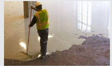
Schönox AP, synthetic gypsum, self-leveling compound, was used for the project. Synthetic gypsum is created from the by-product of the process used to purify emissions from power plants making AP a strong environmental choice as well as floor leveling solution.
