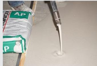
Installation of Schönox AP, synthetic gypsum, self-leveling compound, using a pumping operation, allows installers to efficiently mix product in one location while others distribute the product throughout the area.
