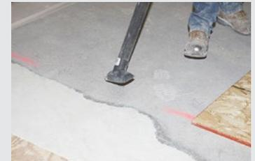
All areas of the renovation space are thoroughly vacuumed with a commercial unit. Removing all dust and debris from the subfloor enhances the bond of the materials to be used later in the project.
