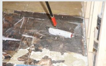
KH Fix was applied from a standing position using a roller and extension rod over a wide variety of wood and residual tile and adhesive residue. The floor was ready for the application of floor leveling compound in under an hour.
