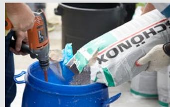
Schönox AP, synthetic gypsum, self-leveling compound, was selected for the project for its superior flow characteristics and ability to be successfully applied to a renovated subfloor with a wide variety of critical conditions.
