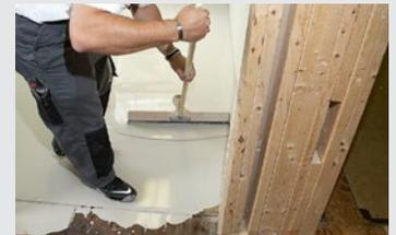
A leveling trowel attached to an extension pole is used to distribute the product and break the surface tension of the compound.
