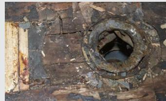
The subfloor surrounding a drain in the floor was particularly damaged, the area uneven, and the substrate brittle.
