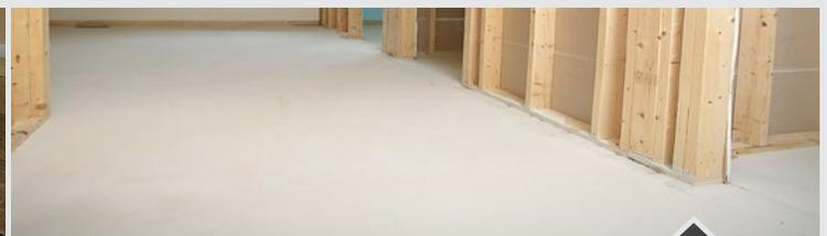
The renovated subfloor will be ready for flooring installation in 24 to 48 hours given the depth of this pour. The product is free of chromates and VOCs and contributes to LEED credits based on its strong environmental credentials.
