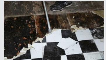
The decision was made to remove this section of sheet vinyl as its adhesion to the substrate was failing. The use of Schönox self-leveling compounds for the project meant that no other tile remnants, glue residue, or wood subfloor pieces had to be removed.
