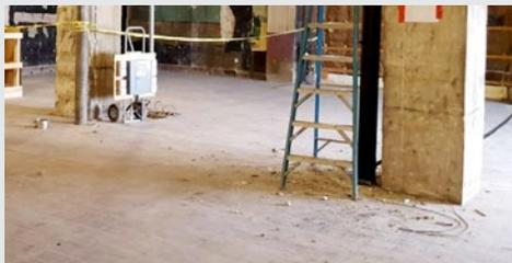
Existing tile, adhesive residue, and uneven substrate conditions required ramping, patching, priming and self-leveling to prepare for installation of a variety of top-surface flooring materials.
