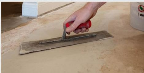
All corridors were troweled with Schönox AST synthetic gypsum rapid-drying, smoothing and patching compound to ramp off the thresholds.
