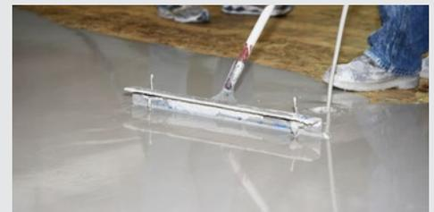
Schönox AP can be installed up to 2" and is ready for foot traffic after approximately 2 hours and covering after approximately 16 hours up to 1/8" layer thickness.
