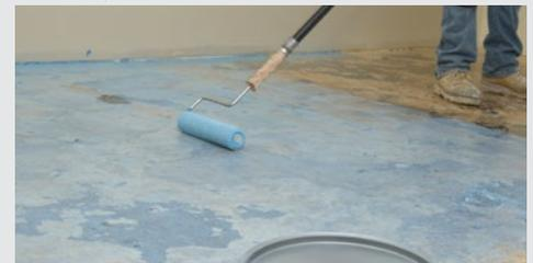
Priming with SHP on the non-porous substrates and using KH Fix to prime and bind residual dust created suitable surfaces for pouring the self-leveler.
