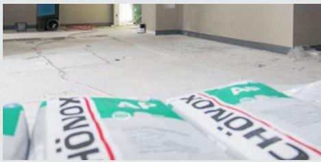
Schönox AP synthetic gypsum self-leveler was used to level approximately 80 percent of the building, including unit bathrooms and bedrooms, common areas and common bathrooms.
