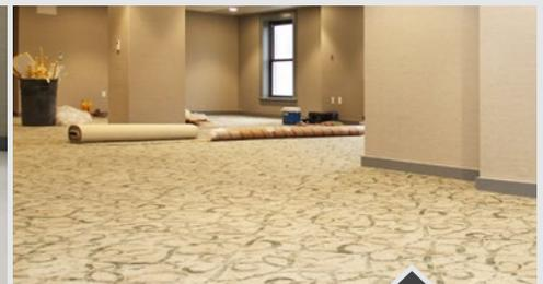
Schönox AP creates an incredibly level, strong and smooth surface, allowing the confident installation of flexible floor coverings. Carpet, VCT and rubber flooring were all installed in the hotel. Over 100,000 square feet of floors of the Hotel Northland have been fully restored using Schönox.
