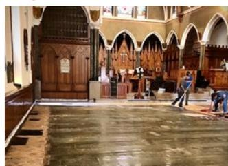
The existing subfloor was cleaned and vacuumed. Poly sheeting was laid over the entire space with its seams fully taped, preventing any liquid subfloor materials used from reaching the underlying church structure.
