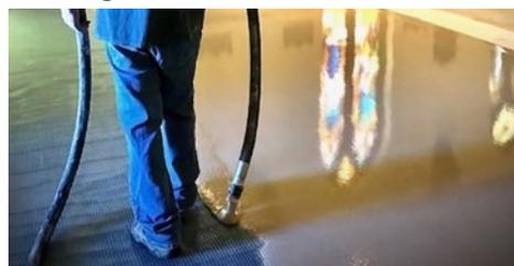
The expanse of the project and the ½ inch intended depth of the pour made pumping of the self-leveling compound atop the Renotex® 3D fabric an ideal project solution for efficiency and consistency.
