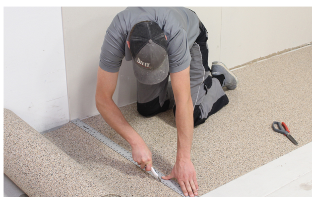
Fig. 3 Roll out material to required length and cut with scissors or utility knife.
