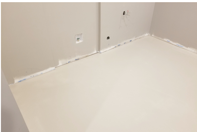
Fig. 10 and Fig. 11 Resin covering coatings.
