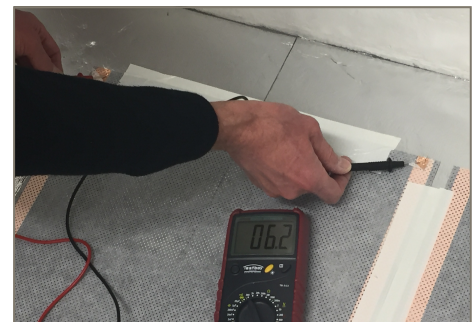
Fig. 8 Measure the electrical resistance of the heaters before application of the covering layer.
