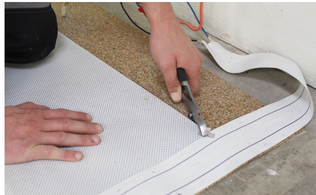
Fig. 4 Locate the heaters and secure in position.
