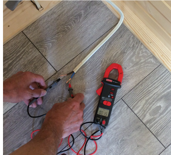
Fig. 9b Measure resistance across the connected power cables after floor covering installation.
