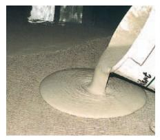
**Leveling over SCHÖNOX RENOTEX®** SCHÖNOX APF is installed using a smoothing trowel or a pump. Despite the use of fibers within APF, it is suitable for use with pumping technology.
