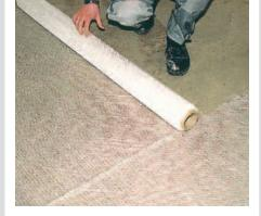
**Laying of SCHÖNOX RENOTEX®** The fabric can be cut with a hook knife. Leave a gap of approx. 1/8" to the walls.
