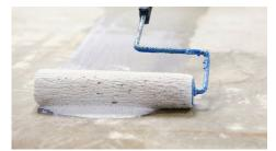
Schönox VD is applied using a 3/8" nap roller.
