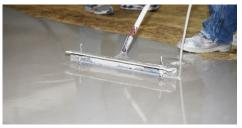
Schönox AP can be installed up to 2" and is ready for foot traffic after approximately 2 hours and covering after approximately 16 hours up to 1/8" layer thickness.
