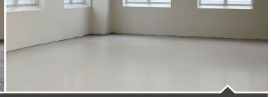
The Schönox AP will be ready for flooring installation in roughly 24 to 48 hours given the depth of this pour. Before the subfloor project, the substrate was not suitable for any floor covering.
