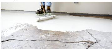
Schönox AP, synthetic gypsum, self-leveling compound flows into the subfloor imperfections with a smooth, efficient consistency.
