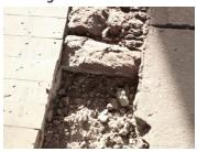
Former dividing walls within the structure presented deeper subfloor imperfections with brick remnants left behind.
