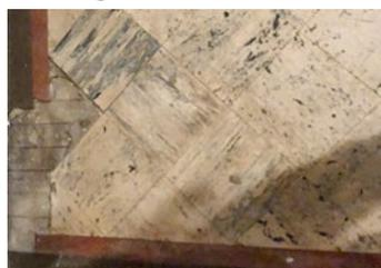
Removal of the carpet floor covering revealed VAT tiles confirmed by lab tests to contain asbestos. The tiles were poorly adhered to the wood subfloor below.
