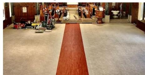
LVT flooring was installed, completing the renovation project with a finished, durable floor with none of the renovation materials adhered to the church's underlying structural surface.
