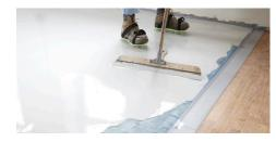
Schönox AP is a synthetic gypsum-based self-leveling compound for the smoothing and leveling of substrates under flexible coverings and wood floors with layer thicknesses of at least 1/8". Designed for interior areas. Schönox AP is suited for:
