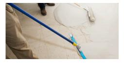
Schönox APF is a fiber-reinforced, synthetic avpsum-based self-leveling compound for wood floors and critical interior substrates. With embedded fibers that make reinforcement fabric unnecessary, Schönox APF can be used on:
