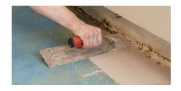
Schönox AST is a rapid-drying, synthetic gypsum-based compound used to provide a very smooth, level finish on various interior substrates. It is suited for:
