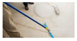
Schönox APF is a fiber-reinforced, synthetic gypsum-based self-leveling compound for wood floors and critical interior substrates. With embedded fibers that make reinforcement fabric unnecessary, Schönox APF can be used on:
