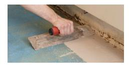
Schönox AST is a rapid-drying, synthetic gypsum-based compound used to provide a very smooth, level finish on various interior substrates. It is suited for:
