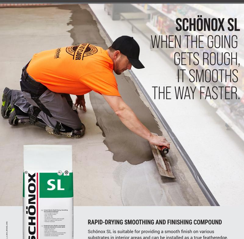
substrates in interior areas and can be installed as a true featheredge. With its moisture-resistant characteristics, Schönox SL can prevent flooring installation failures due to loss of adhesion when paired with a moisture-resistant adhesive.
